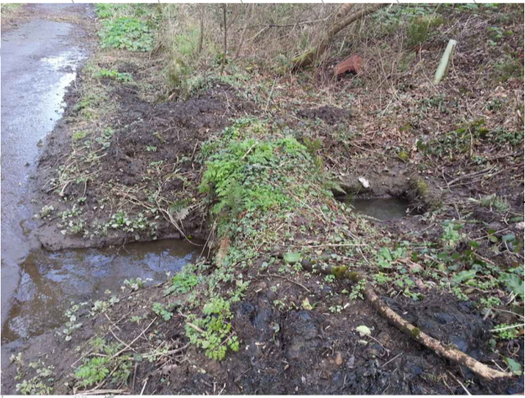
Photo 4 - Piped under track, outfalls to short open ditch and then to open catchpit. Outfall from catchpit piped towards highway culvert
