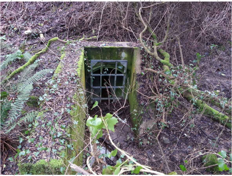
Photo 6 - 900Ø highway culvert (passes beneath A390)
